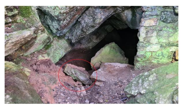
The boulder was "Plugged and Feathered" into manageable pieces and stacked out of the way. A follow-up inspection two weeks later revealed no further issues.
